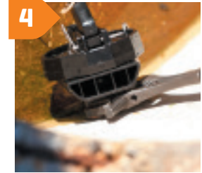
Valve body is suitable for final tightening with a wrench/multigrrips to ensure valve is perpendicular.
