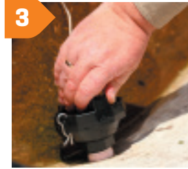
Screw the float valve into the trough inlet, using the body, by hand until tight.
