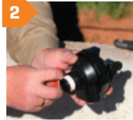
Apply PTFE Tape in clockwise direction, ensuring thread is adequately covered.
