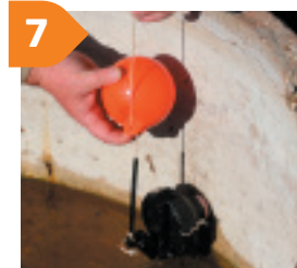
Check float position against side of trough.
